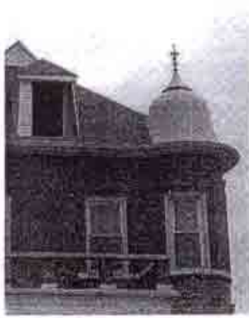
A house under restoration
